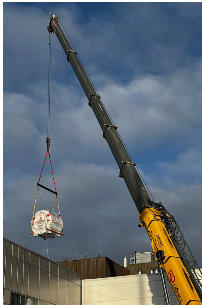
Pictured: Crane owned by Cherubini Group, lowering DGH's new MRI into the hospital through the roof on Dec. 22, 2023
